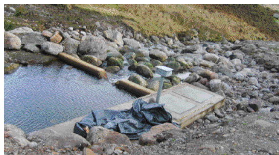
The weir on the Mahon River which provides Mahon Hydro turbine with water.
