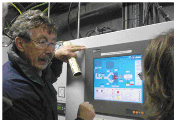
Sean Murphy explaining how the hydro turbine works.
