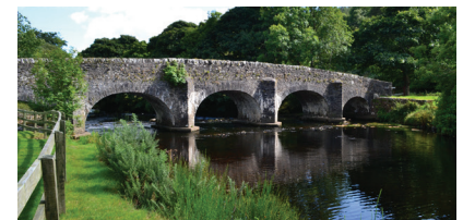
The 18th century bridge at Clara Vale
