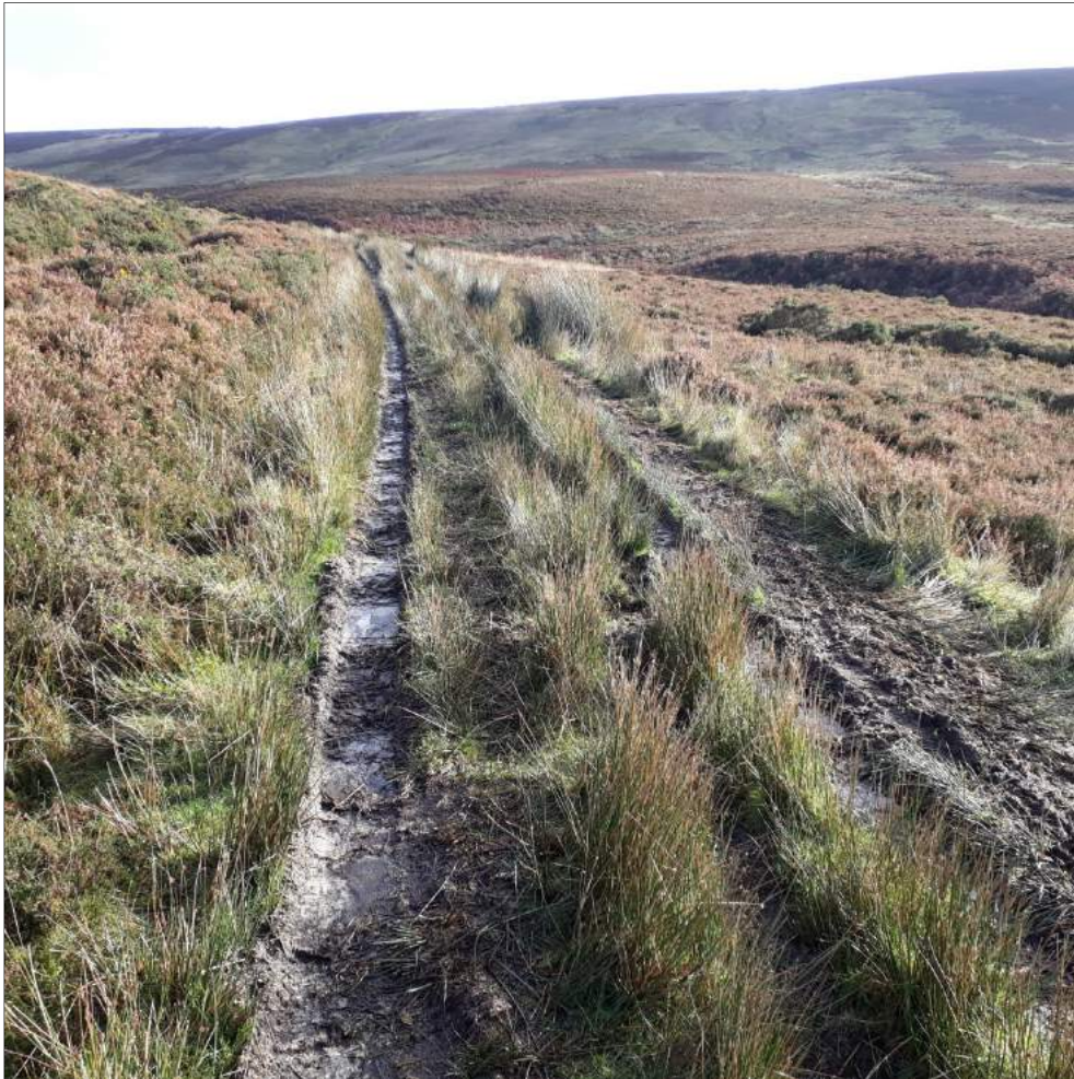
Plate 2. Tyre tracks have created deep channels for water to flow down on the track above the old borrow pit.
